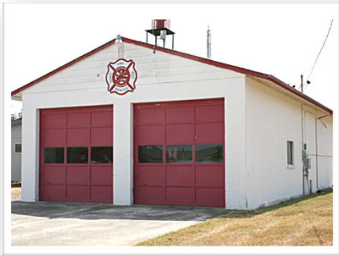
Figure 7: Station 35 - 121 Sunshine Ave.
