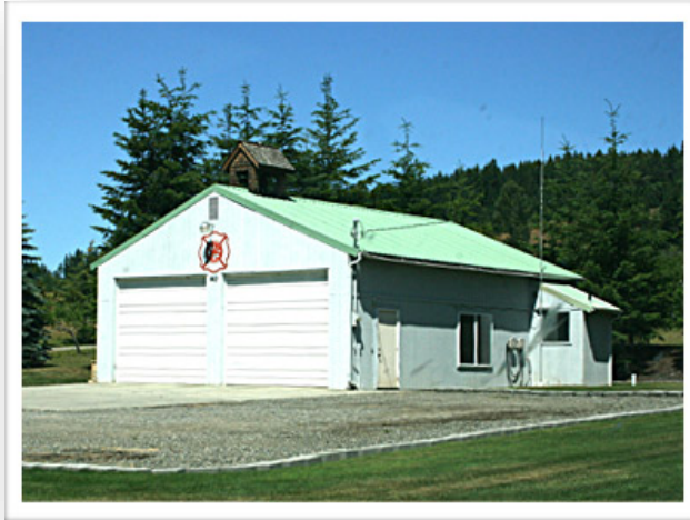
Figure 8: Station 36 - 40 Texas Valley Road
