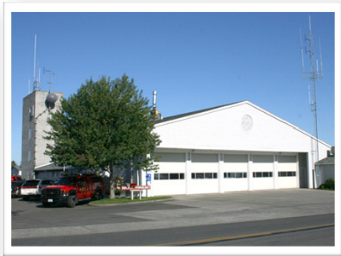
Figure 6: Station 34 - 323 N. 5th Ave.
